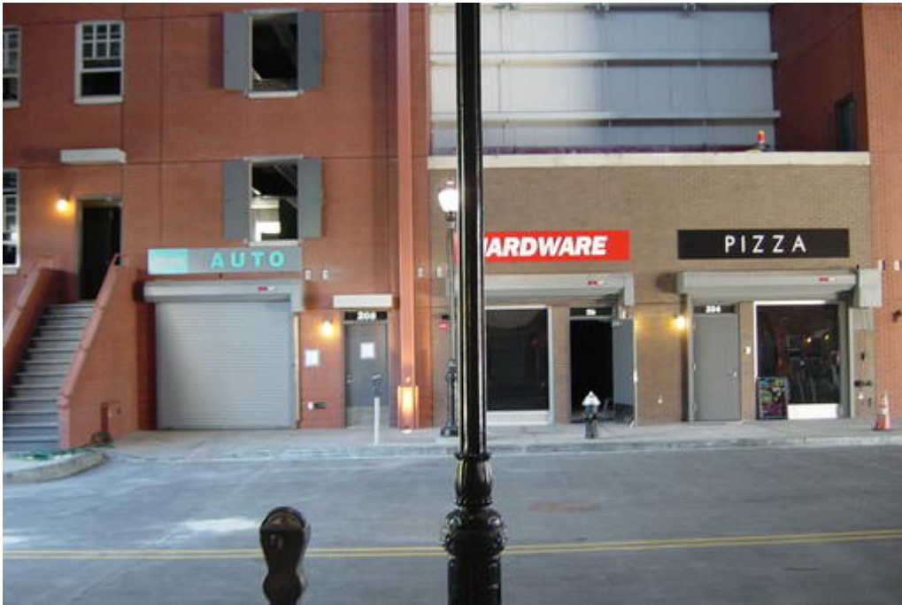
Figure 1. The NYFD Training Facility at Randall's Island
